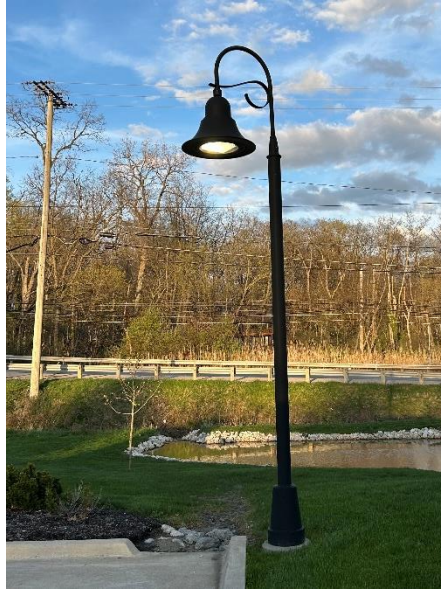
Figure 604-B – Cut-off light fixture example
